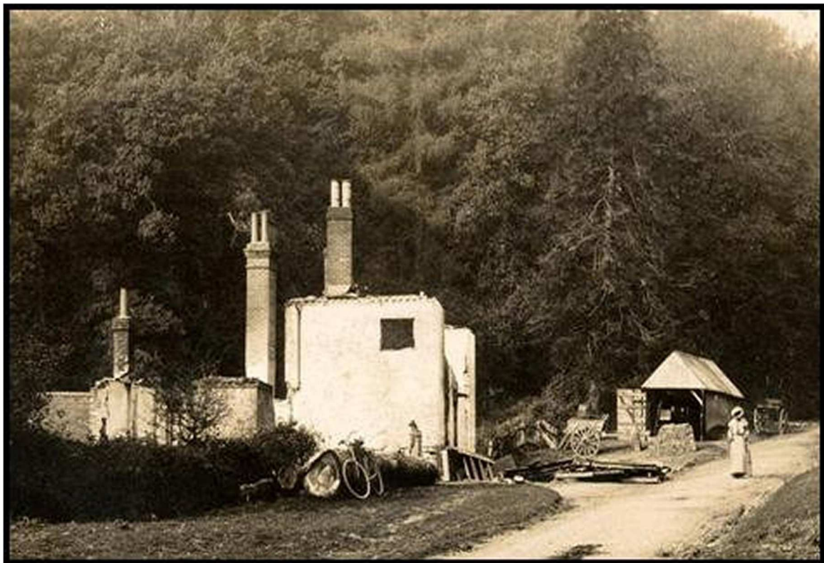
The original Windmill Inn, Pitch Hill, after the 1906 fire
